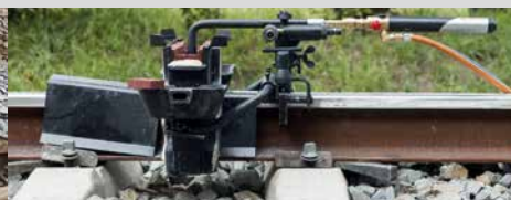
SMARTWELD RECORD Documentation of the preheating process
