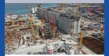
Location: Senegal Client: EIFFAGE GENIE CIVIL Caisson size (m): 28 x 55 x 28 Caisson weight (ton): 16 700 Total number of caissons: 21 Scope of Works: Heavy Duty Slipform and Transfer
