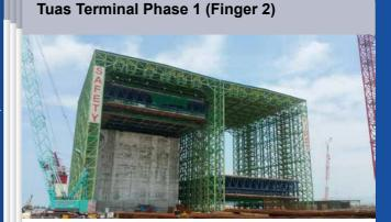
Location: Singapore Client: DAELIM INDUSTRIAL CO.LTD Caisson size (m): 28 X 40 X 28 Caisson weight (ton): 15 200 Total number of caissons: 221 Scope of Works: Gantry Slipform and Transfer
