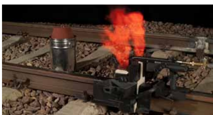
THERMITE WELDING
